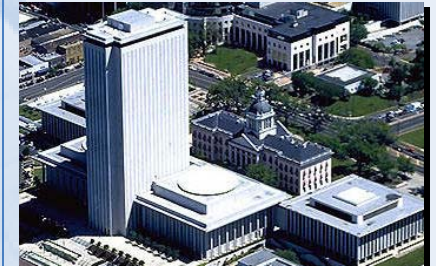
The Capitol Building - Tallahassee, Florida
